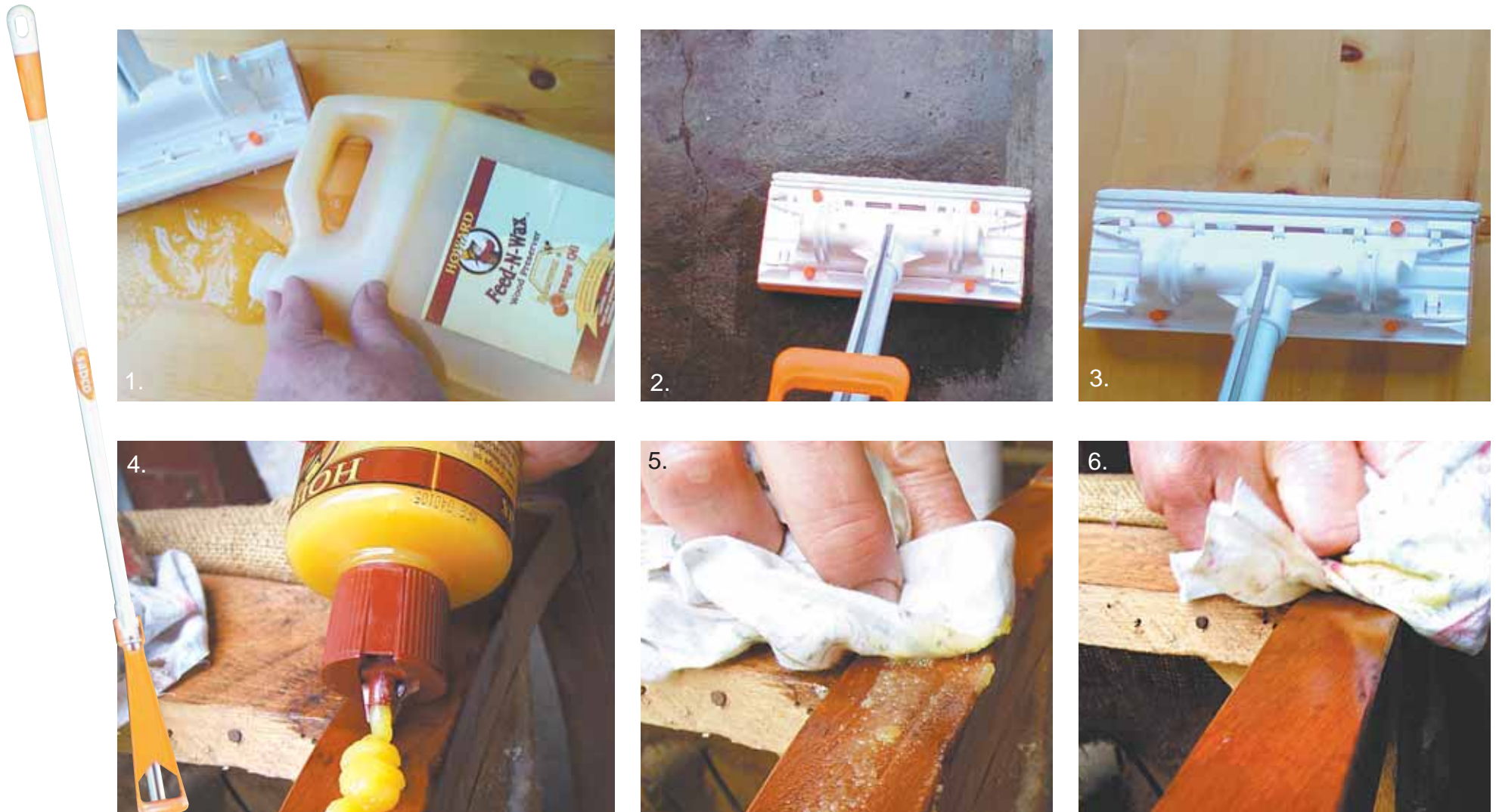
1. Squeezing Feed-N-Wax on the floor 2. Mopping onto concrete 3. Mopping onto floorboards 4. Squeezing Feed-N-Wax on to furniture 5. Spreading Feed-N-Wax with a soft cloth 6. Buffing the furniture
